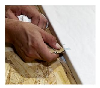
Sand excess bondo\* following the shape of the area. Clean the area with alcohol before proceeding with paint.
